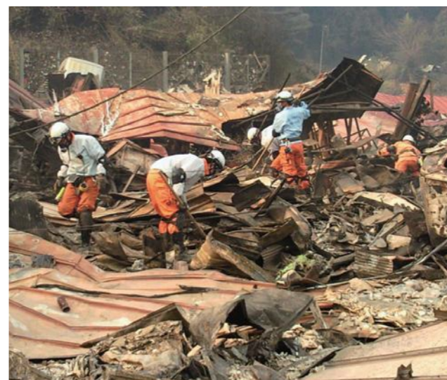
東日本大震災の被災地における緊急消防援助隊の活動 Emergency Firefighting Support Team in a disaster-affected place in the Great East Japan Earthquake and Tsunami
